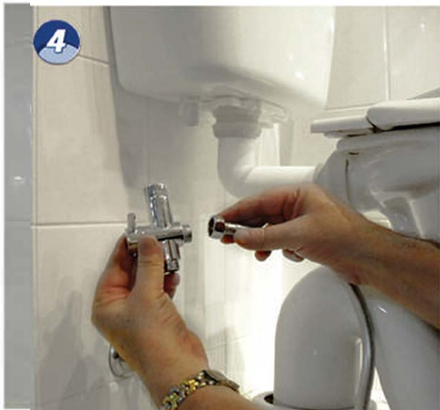
4 Fit handspray hose to water diverter, ensuring you insert black washer.
