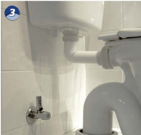
3 Place dual check on tap, ensuring you insert into the bottom of the backflow dual check.
