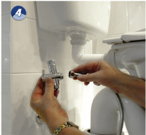
4 Fit handspray hose to water diverter, ensuring you insert black washer.
